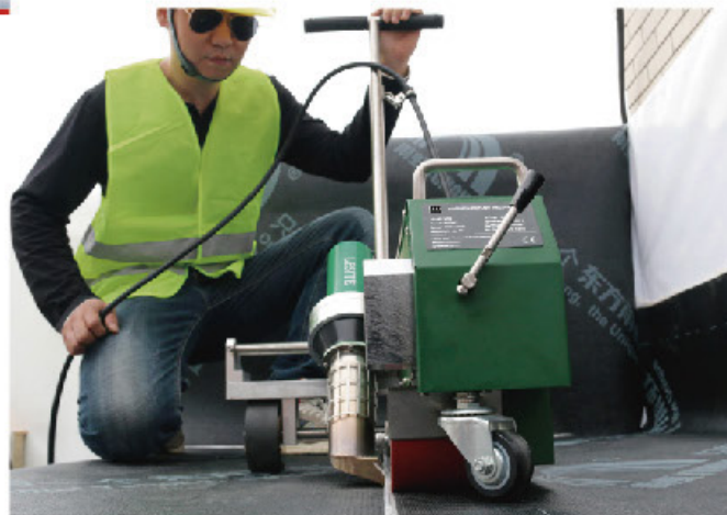
Welding Modified SBS by Flameless Method LST-WP2
